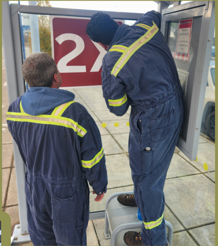
Fleet employees Scott Wright and Jose Mora-Manzo installing graphics
