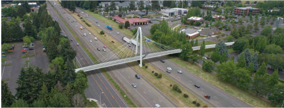
Figure 4 Isometric View of the Cable-Stayed Alternative
