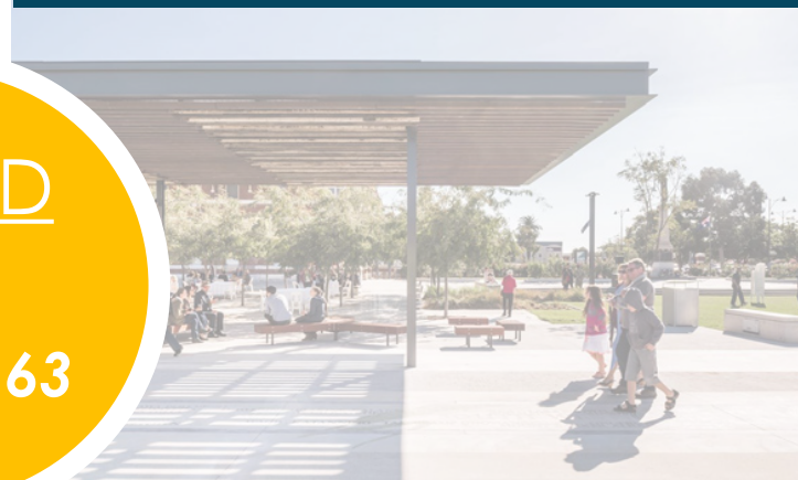
Open Shade Structure
