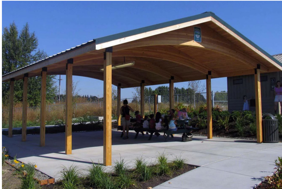
picnic shelter - Western Wood Structures treated Douglas fir, powdercoated steel (dark green), standing seam metal roof (dark green)
