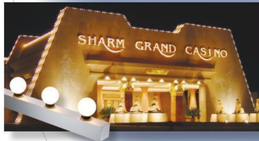
EXC Series wired for four-channel chase dramatically highlights the contours of this casino perimeter.
