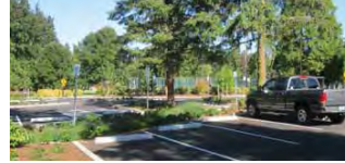
Existing Parking Lot
