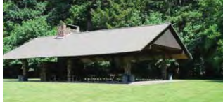
Existing River Shelter
