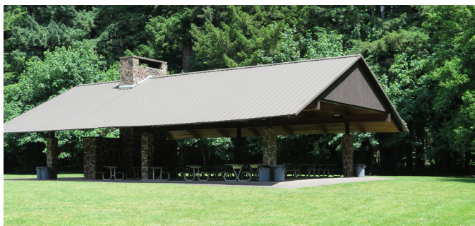
Existing River Shelter
