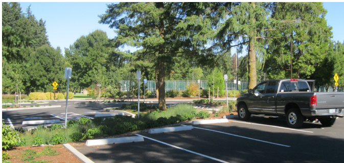
Existing Parking Lot
